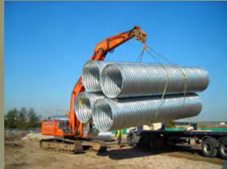
1400mm Ø pipe bundle (30m) weighs less than 2.0t
