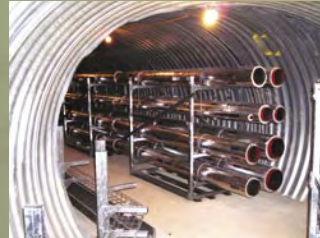
2.80m Ø service tunnel
