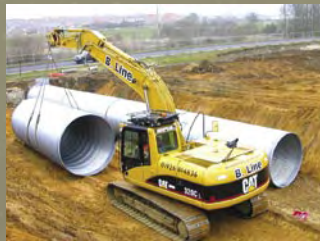
3.0 mtr dia culvert, 120mtrs installed in two days
